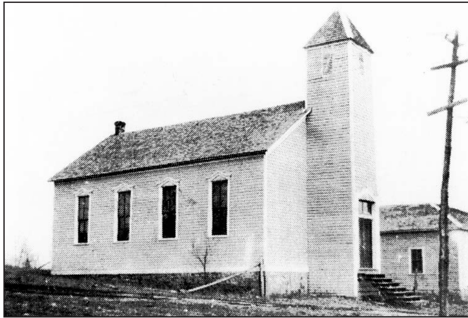
Vienna Methodist Church, ca. 1914, was built in 1885. According to local historian John Viessman of Vienna, the building is sitting on log sleepers, which is one side of the log flat and the rest round. The perimeter logs were hued square. Photo courtesy of Vera McDaniel Jones.
