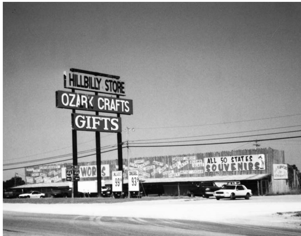
The last section of I-44 completed in Pulaski County bypassed the four-lane through Hooker Cut. Sterling moved to the Highway 28 overpass. Photo courtesy of Sterling Wells.
