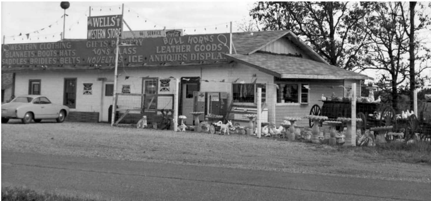
Dallas and Joyce Wells, Sherry's parents, had a Western Store on Route 66 during the 60s and 70s. It was located at the Buckhorn. This building was razed for the construction of the I-44 Buckhorn overpass and a small strip mall was built. Sterling's last store was located in one of the buildings. Photo courtesy of Sherry Wells Ernst.
