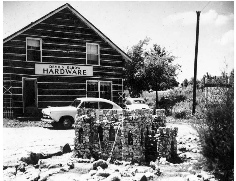
Mr. Tarbell had a hardware store on the first floor of Hiawatha Lodge in Devil's Elbow for a short time. In the foreground is Uncle Cummy's rock castle under construction.
