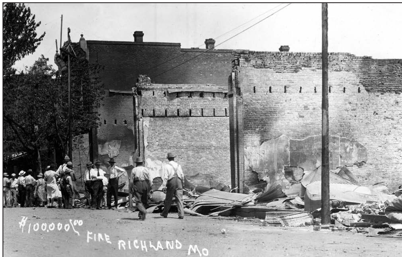
The scene that sparked our interest in Richland's big fire also led to Richland's interest in building a municipal water system when the smoke cleared. This appears to be the first fire of the business row along McClurg Avenue. Courtesy of Jan and Terry Primas.
