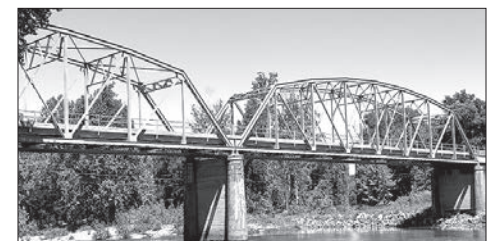
View of the two-span Parker through truss bridge at Devils Elbow.
